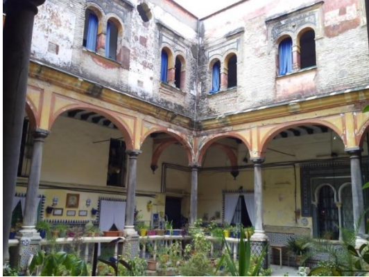
Image 1. View of Pumarejo Palace
